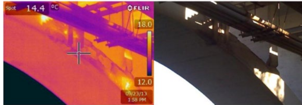
Figure 3: Upstream: Arch delaminations around pipe bracket and corners
